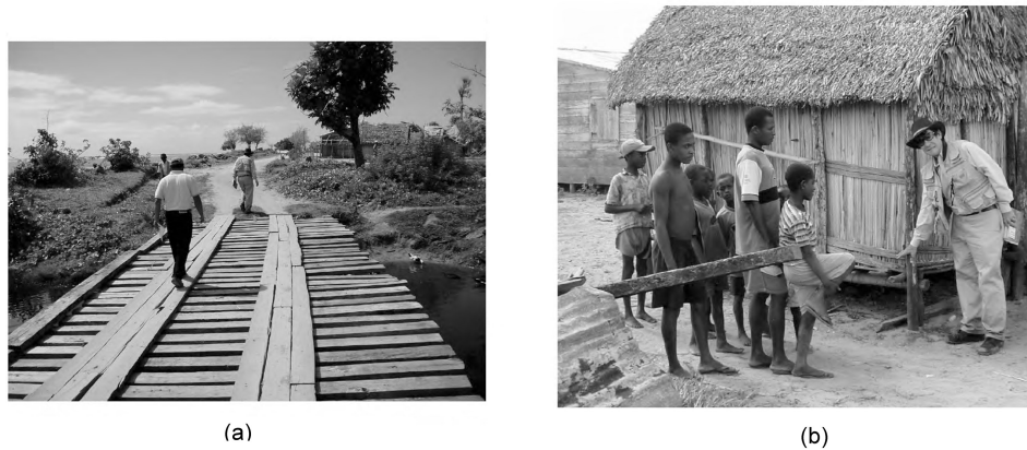
Figure 4. (a) The road bridge at Ambodihampana (Site 2), looking south toward a village. The former bridge at this location (described by witnesses as “equivalent” to this new one, rebuilt since the tsunami) was carried away by the waves during the tsunami. (b) The water reached a height of 50 cm inside the houses of the village, corresponding to a total runup of 2.5 m, for an inundation of 80 m.
