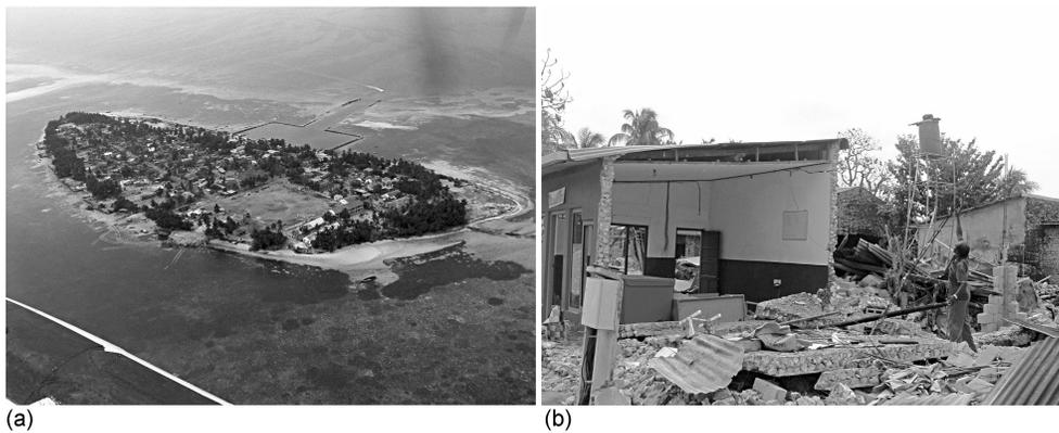
**Figure 4.** Vilufushi Island (Thaa Atoll): (a) southwest view with the harbor toward the inner portion of the atoll, as seen during the landing approach from a seaplane; (b) classic blowout failure of a coral stone wall.
