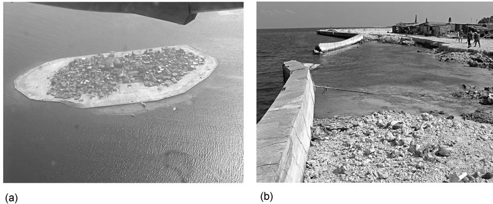
**Figure 10.** Kandholhudhoo Island (Raa Atoll): (a) eastward view of the island from the air; (b) collapsed seawall with exposed armor on the northwest side of the island.
