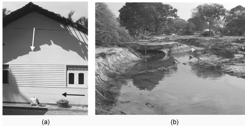
**Figure 12.** (a) Weligama: a partially destroyed building. Note the nearly vertical crack on the wall that faces the sea (white arrow) and the standing-water mark (black arrow). (b) Yala: back-wash scour of foundations.
